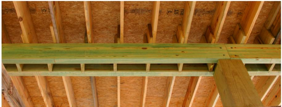
Shown during construction, treated glulam beams are set on piers to support the floor system above.
