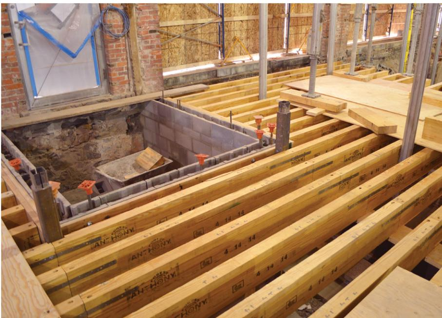
The floor is framed with 20-foot, 3-1/2-inch-by-9-1/2-inch glulam beams spaced 12 inches on center.
