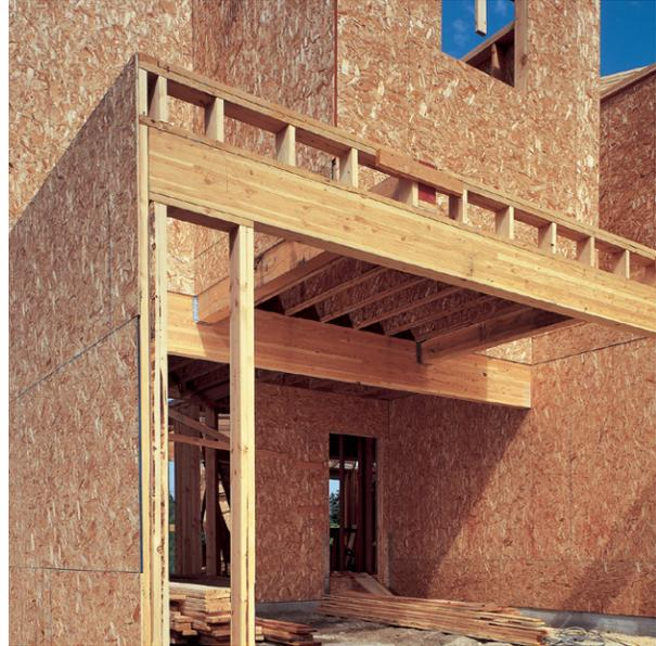
**The ability of glulam beams to span long distances and their dimensional stability makes them an ideal option for garage door headers.**
