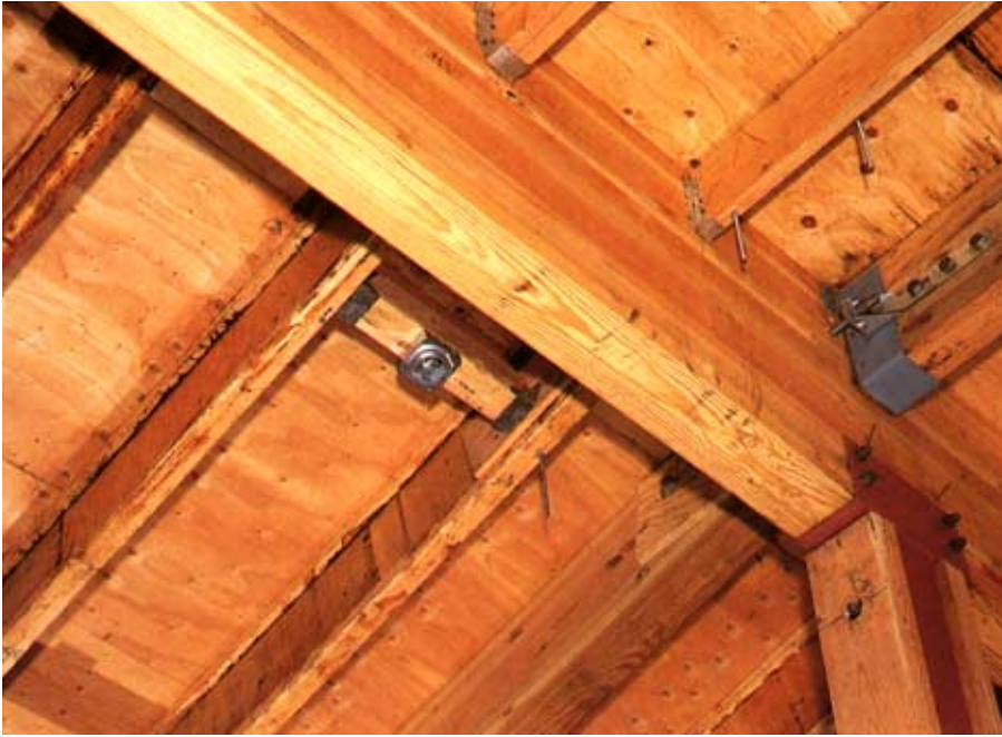
The use of APA trademarked glulam beams, I-joists, and plywood sheathing create a cost-efficient campus.
