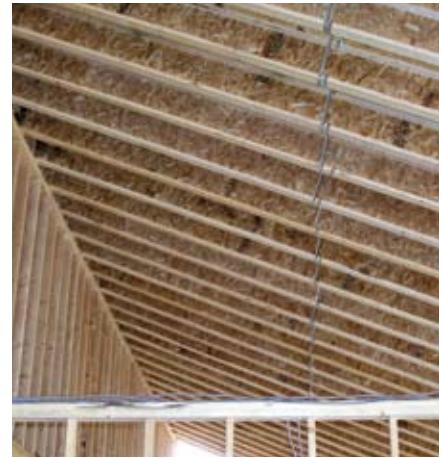
APA trademarked 14-inch-deep I-joists were used for the school's rafters.
