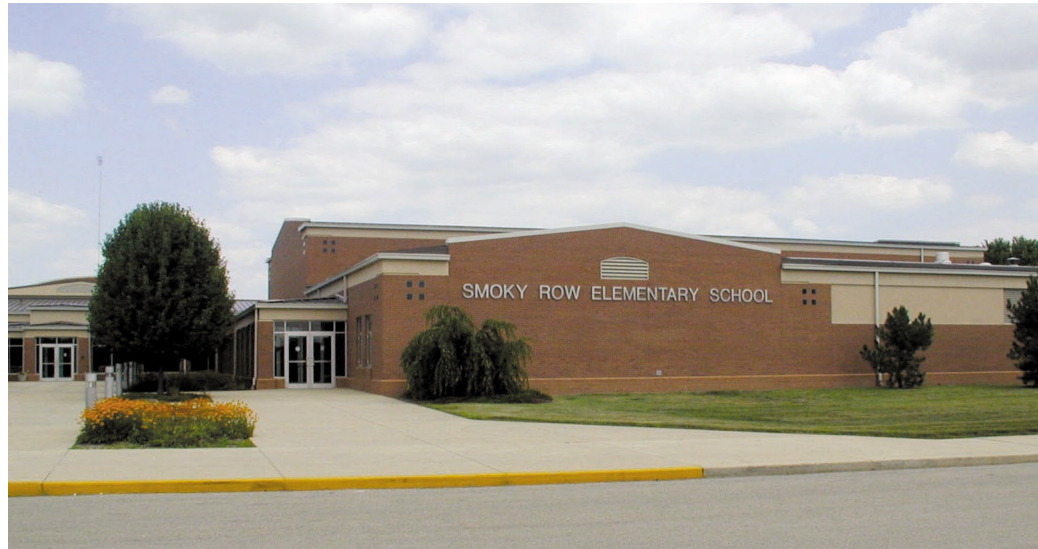
Architects featured exposed glulam trusses and laminated wood decking in the cafetorium and media center of Smoky Row Elementary School in Carmel, Indiana.
