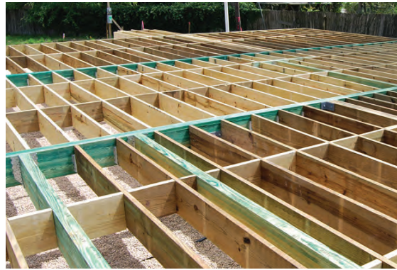
Raised Floor Construction
