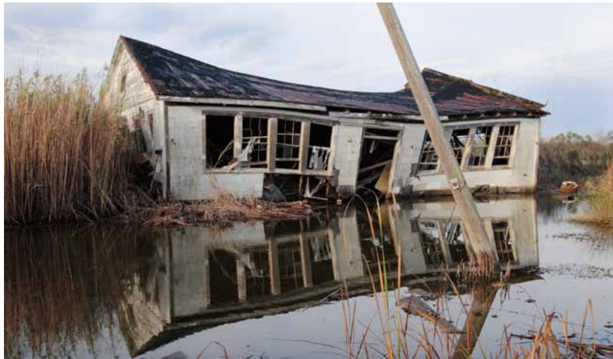
A house lifted off its foundation and destroyed by Hurricane Katrina, Irish Bayou, New Orleans, Louisiana
