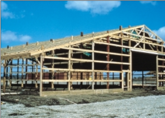
Large wall openings are possible with wide post spacings.
