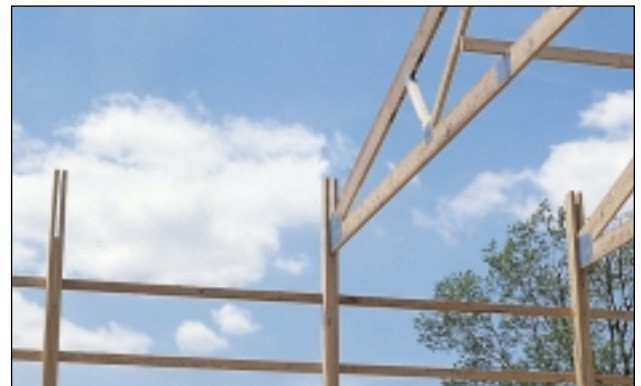
Truss to laminated column connection.
