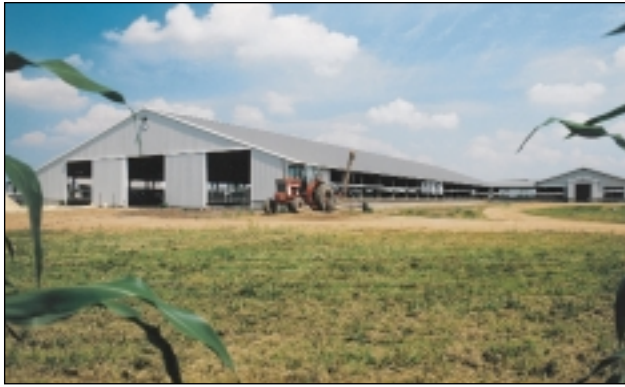
Post-frame designs incorporating diaphragms and shear walls reduce post size and embedment requirements.
