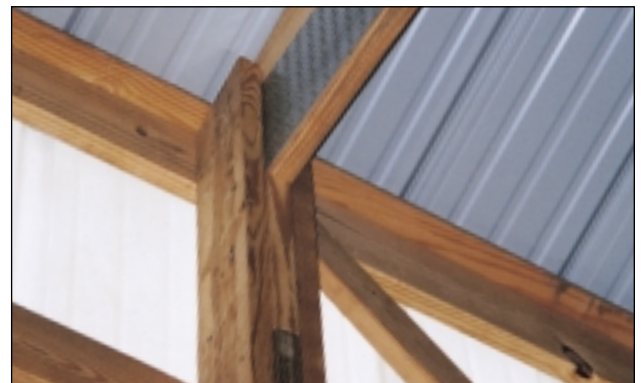
Closer view of a truss to laminated column connection.
