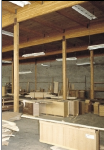
Solid-sawn columns used to support glulam beams.
