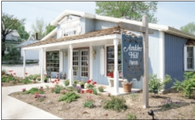
T-111 plywood-sided commercial building.
