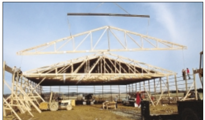
Erection of long span trusses.
