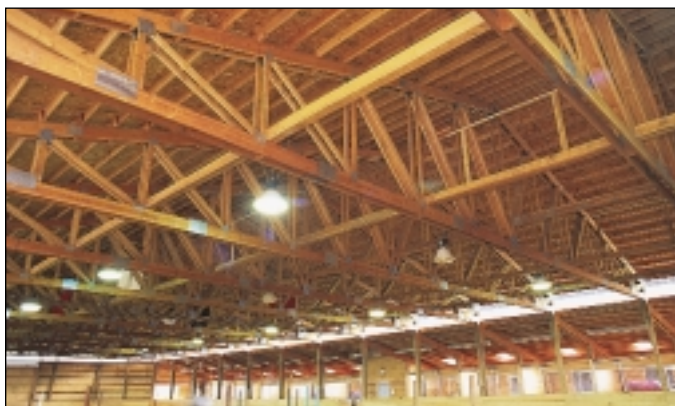
Post-frame construction allows for an open 72-foot span in this equestrian facility.
