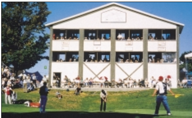
These viewing stands used diaphragms and shear walls to transfer lateral loads.
