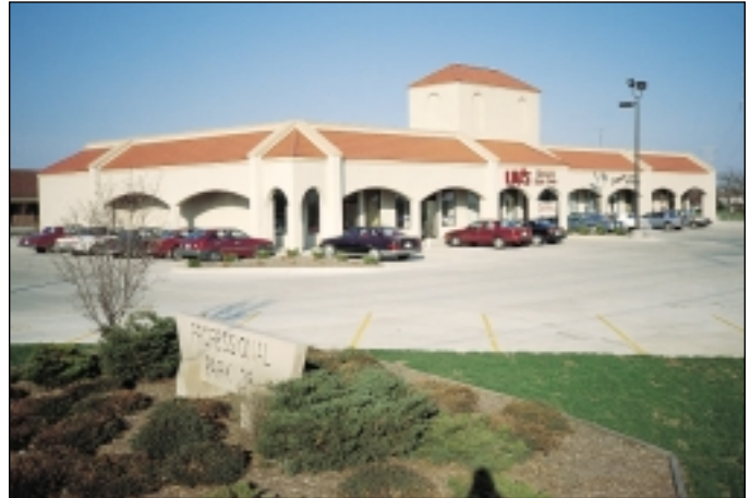
Post-frame commercial occupancy.
