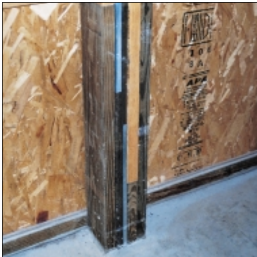
Treated nail-laminated post.
