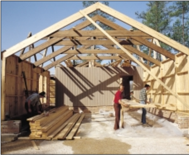
A small commercial building using rafters.
