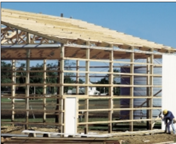
Horizontal wall girts supporting sheathing.
